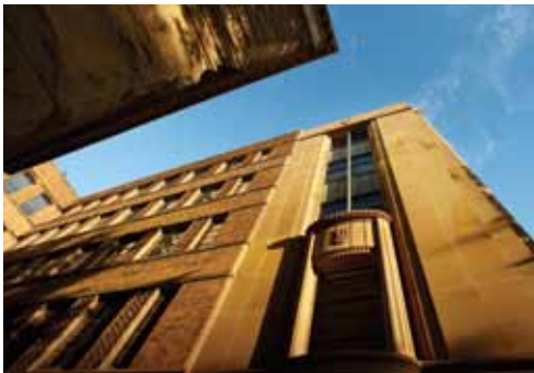
99 Macquarie Street, in the heart of Sydney CBD, is home to Mulpha Australia Limited.
