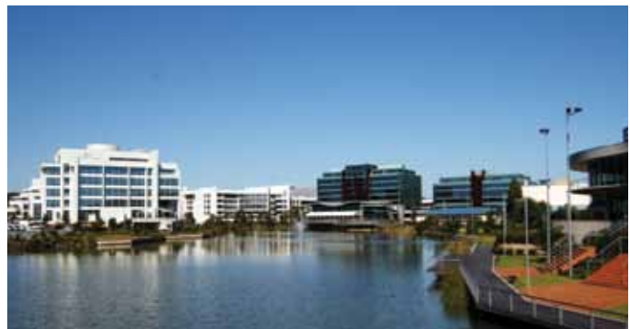
The 377-hectare world-class Norwest Business Park located at Baulkham Hills in the northwest sector of Sydney, New South Wales.
