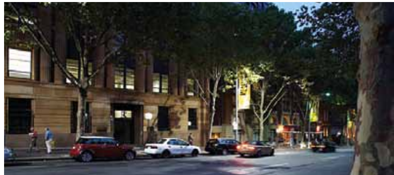
99 Macquarie Street, originally known as Transport House, was built in 1938 for the New South Wales Department of Motor Transport. This classic art deco building has undergone a complete A$30 million refurbishment by Mulpha Australia and is now one of Sydney's most prestigious business addresses.
