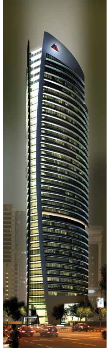
Menara Mulpha, a 30-storey grade A office tower, is designed by the world-renown New York architect, Kohn Pederson Fox.
