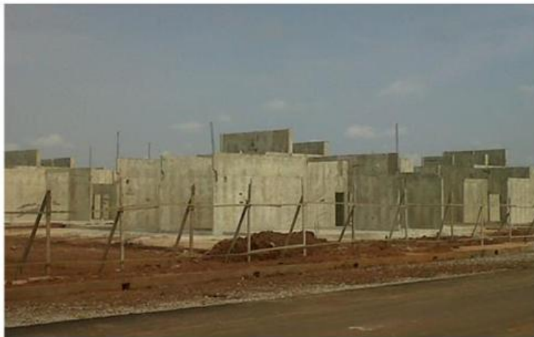
Figure 18: Product after IBS prefabricated components removed
