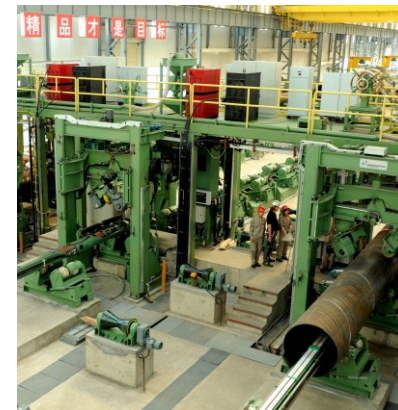
Zhongyou BSS new production facilities are now in full production
