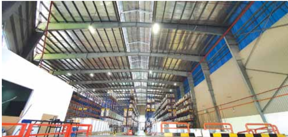
[Courtesy by RMSB – LED lightings inside the warehouse (partially)]
