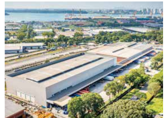
Pasir Gudang Logistics Warehouse 2
