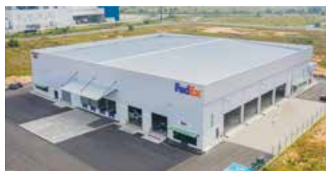
AXIS FACILITY @ BATU KAWAN GreenRE 铜级认证
