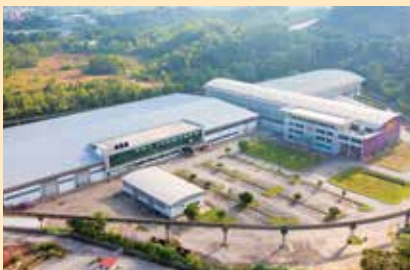
AXIS INDUSTRIAL FACILITY @ RAWANG
