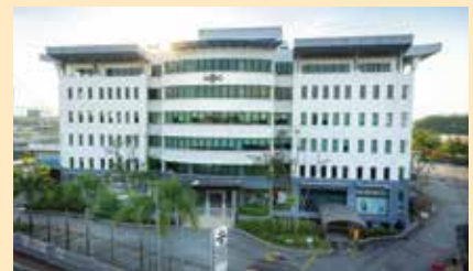
AXIS TECHNOLOGY CENTRE
