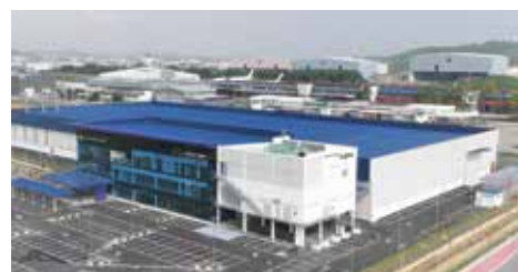
AXIS AEROTECH CENTRE @ SUBANG GreenRE 铜级认证
