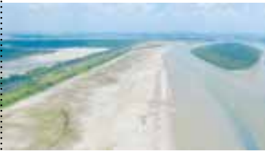
Land reclamation for Pulau Indah, Port Klang
