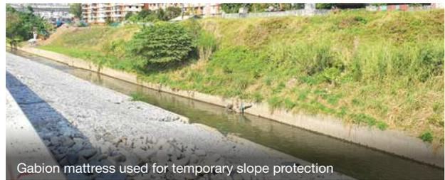
Gabion mattress used for temporary slope protection
