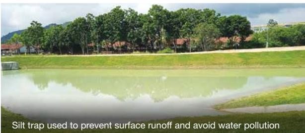
Silt trap used to prevent surface runoff and avoid water pollution
