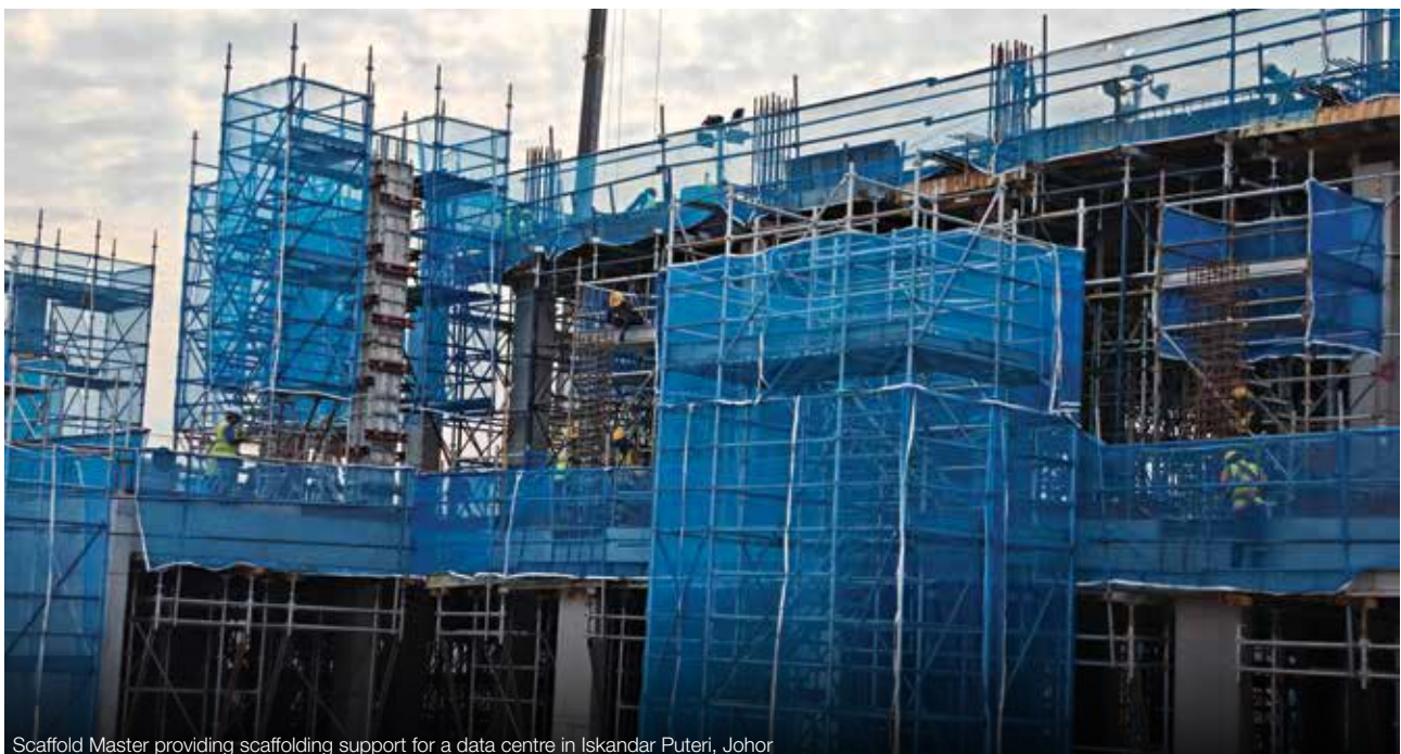
Scaffold Master providing scaffolding support for a data centre in Iskandar Puteri, Johor
