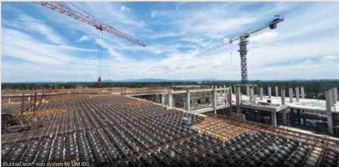
BubbleDeck® slab system by IJM IBS
