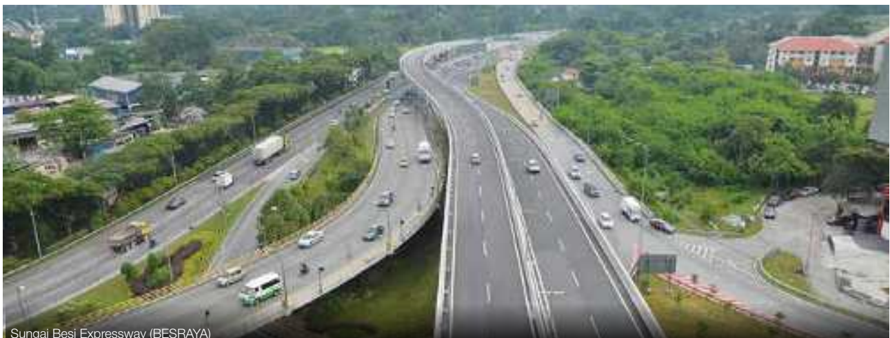
Sungai Besi Expressway (BESRAYA)
