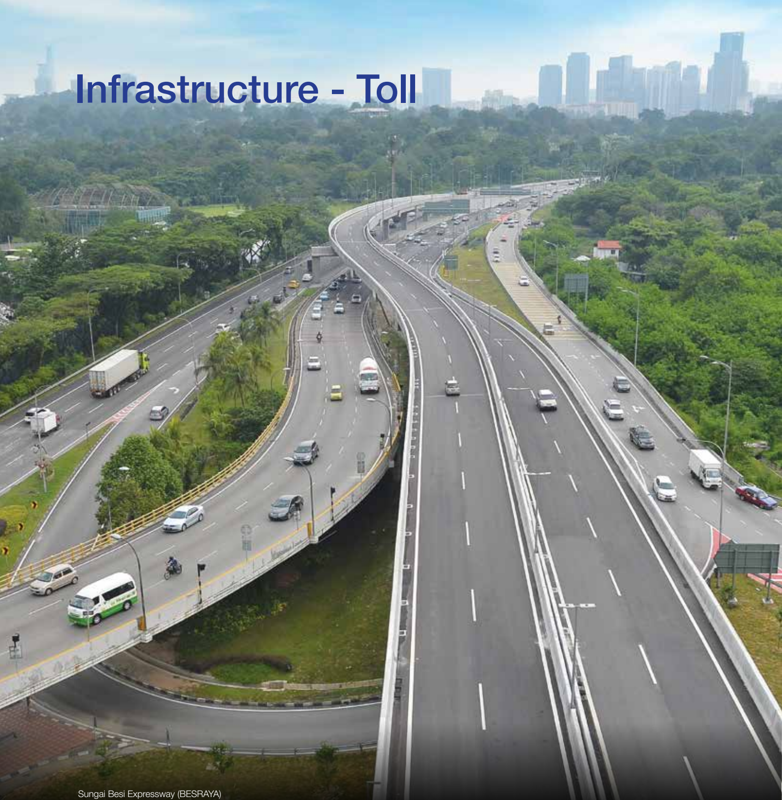
Sungai Besi Expressway (BESRAYA)
