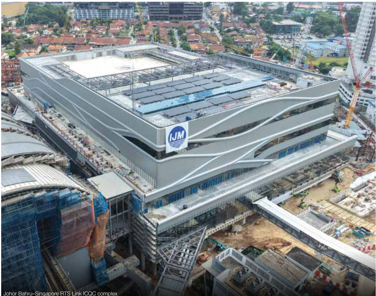
Johor Bahru-Singapore RTS Link ICQC complex
