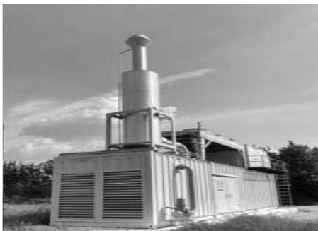
Biogas / landfill power plants use methane gas produced by decomposed organic waste and/or wastewater as combustion fuel to spin the turbines to generate mechanical energy which then activates the generator to create electrical energy.
