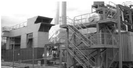
Combined cycle plant produces electrical energy using natural gas and steam. Natural gas is burned to create heat. Heat spins the gas turbines to generate mechanical energy which then activates the generator to create electrical energy. The waste heat released from the gas turbines is captured to generate steam which is used to generate more electrical energy.
