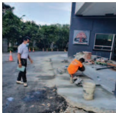
Upgrade in progress
