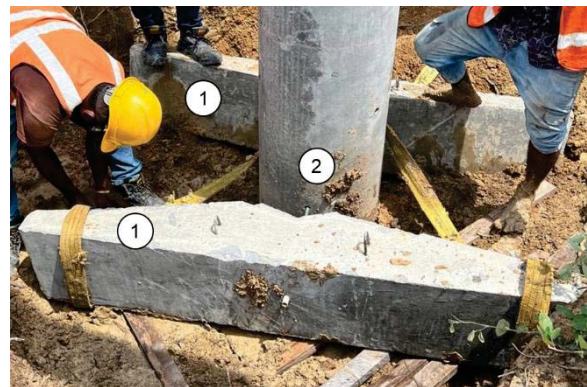
Our concrete kicking blocks (1) secured to a standard pole (2)
